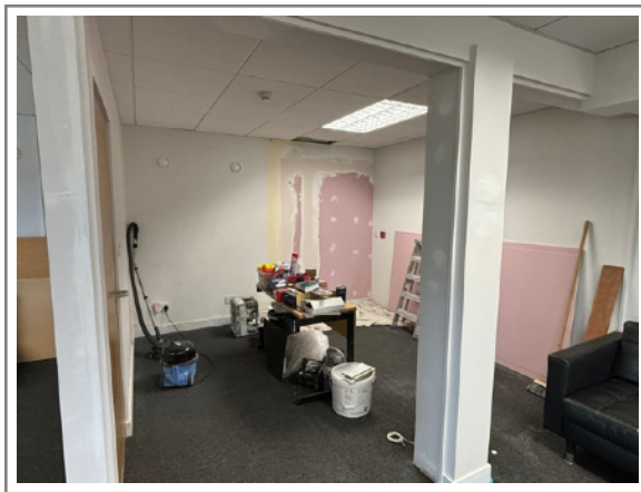
Work in progress blocking the old access door to CIASL
